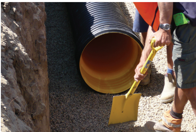
Granular material spread evenly in the trench
