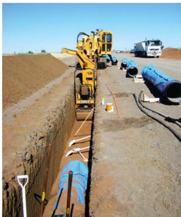
DN450 Irontite® pipe in typical trench with blue sleeving for water supply pipeline
