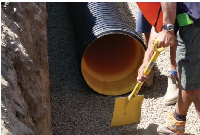
Granular material spread evenly in the trench
