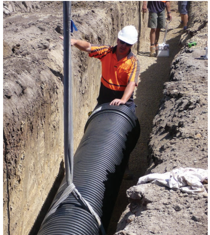
BlackMax pipes lowered into the trench with a nylon sling
